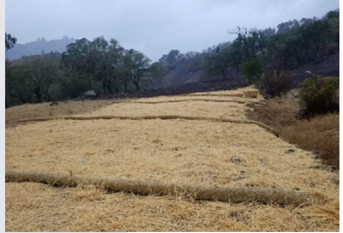
Loose straw mulch and straw wattles are among the methods used to prevent soil erosion and debris runoff at Kimball Reservoir following the Tubbs Fire. Photo from Calistoga Public Works Staff
